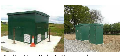
Indicative Substation and gas governor enclosures
